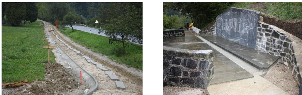
Sliki 7 in 8: Obnova spominske ploščadi in poti
