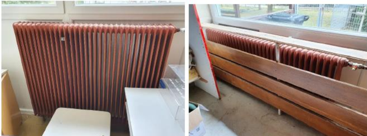
Slika 36: Radiator z navadnim ventilom in radiator s termostatskim ventilom
